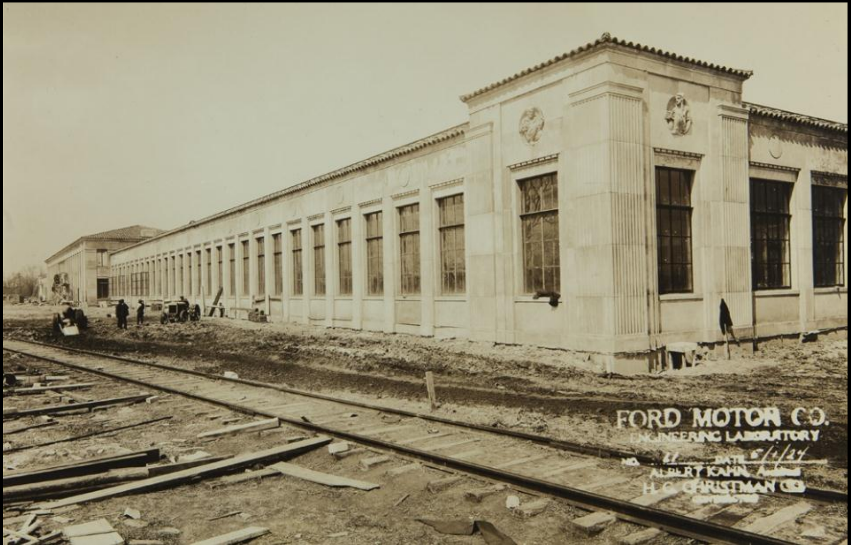
Again a photo from the original construction of the building. The exterior beauty of the building is attributed to the materials used for construction. The facing material is Bedford Limestone from Indiana and the roof has a very distinctive look with red clay shingles.
