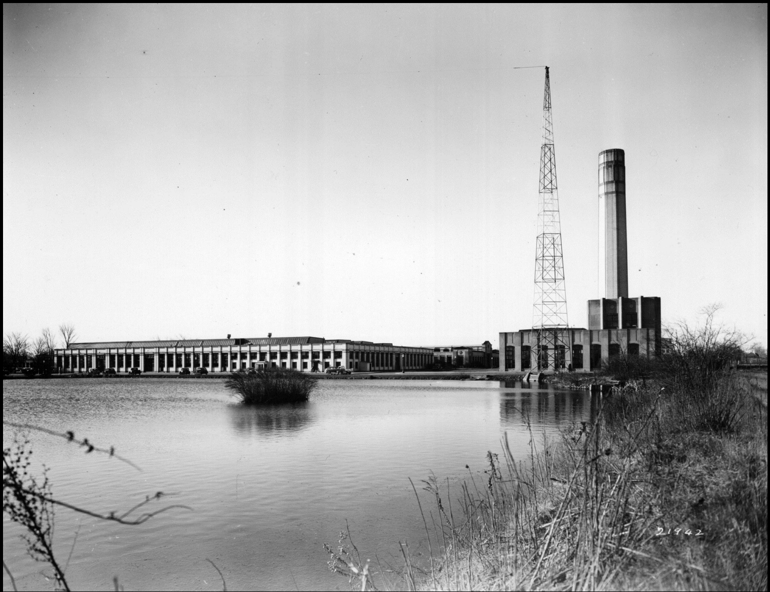
Rear View of FEL from Greenfield village
